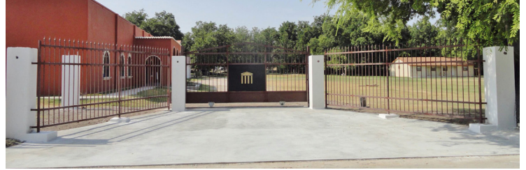
THE COMPLETED ENTRANCE GATE
