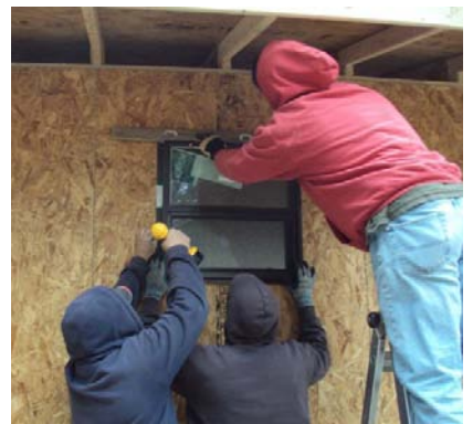
Indiana Work Group. Compass Team working on Duplex #5 for married students. Colleyville men installing windows on Duplex #5.
